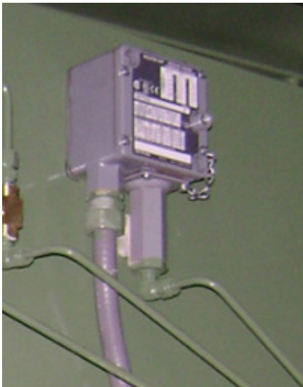
FIGURE 11- HIGH AND LOW FLUID PRESSURE SWITCH
