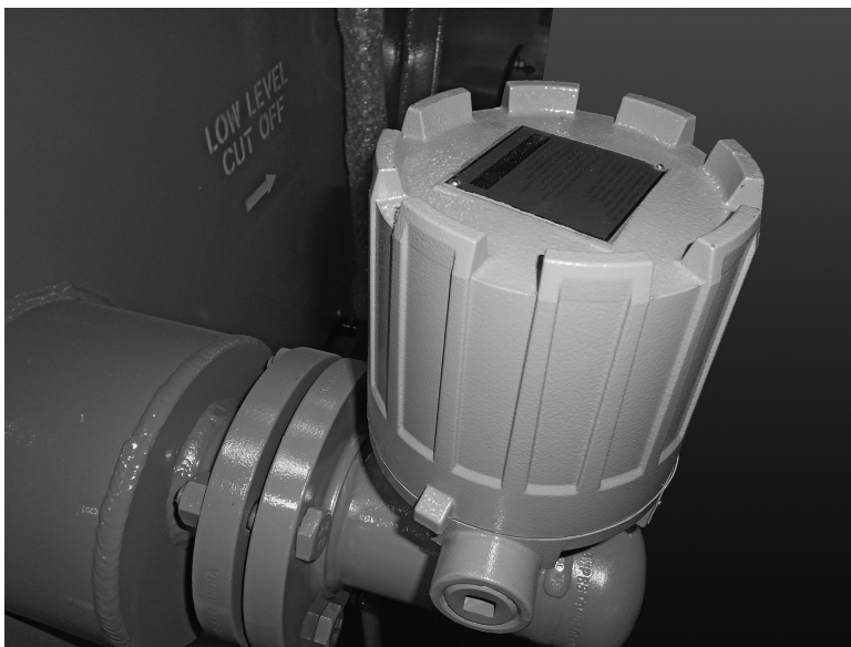
FIGURE 9A - LIQUID LEVEL SWITCH LOCATION
